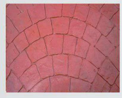
Stampcrete System is cast-in-place concrete, integrally colored and stamped with texturing tools to produce a surface similar to natural stone, brick, slate and other paving materials.
